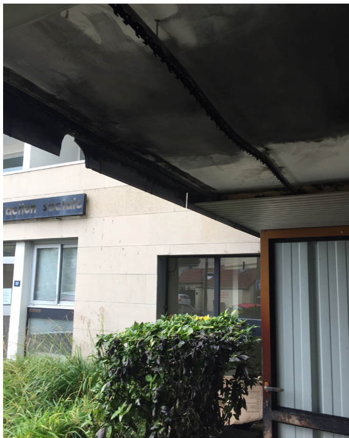
Figure 10: Resultant damage from arson attack on CAMOIE in Rouen.
